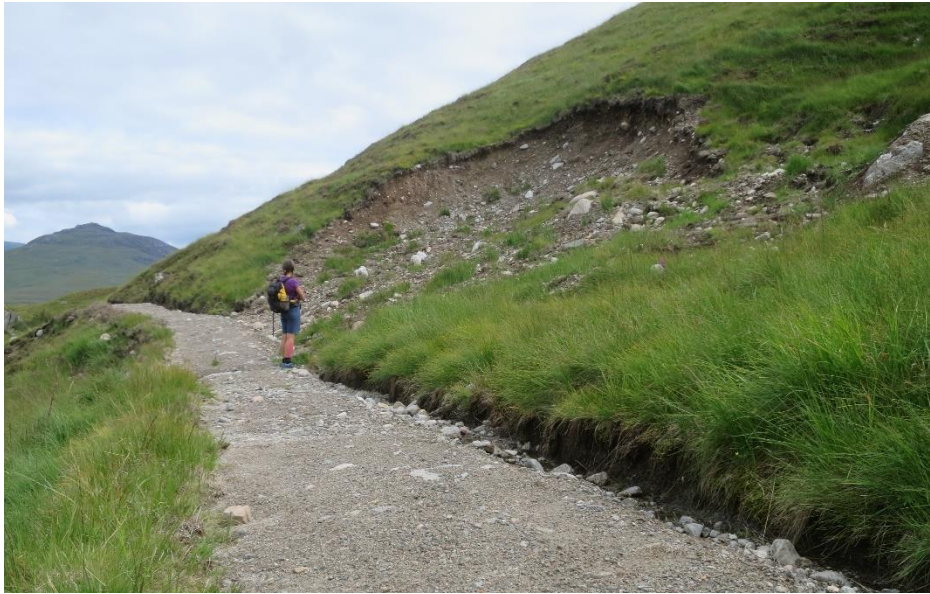
Borrow pit by recently-constructed track, summer 2018
