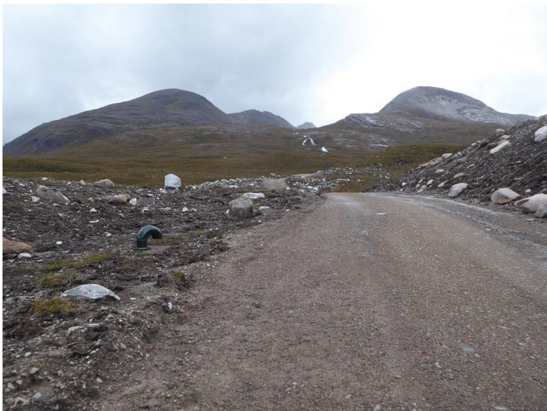
Easan Dorcha hydro scheme, Achnasheen, September 2018(Wester Ross National Scenic Area and Wild Land Area 26: Coulin & Ledgowan Forest) – planning conditions specify that the tracks should be reduced to 2 metres and the ground to the sides restored, not yet carried out
