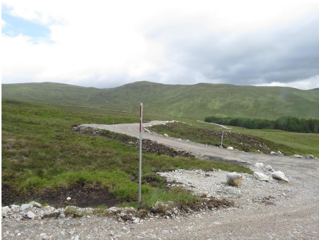
Stronelaig wind farm connection construction track, permission granted for permanent retention (upper sections in distance to be reduced to ATV track). Photo taken June 2018
