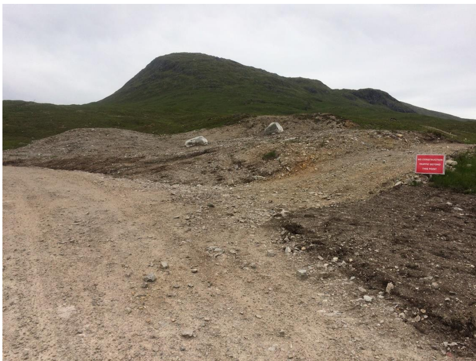
Current impacts of hydro construction near Attadale, Wild Land Area 24: Central Highlands, where four schemes are under construction/have recently been constructed
