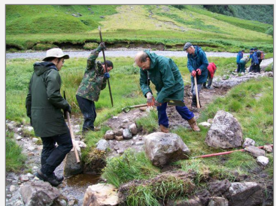
JMT volunteer team working on path improvements
